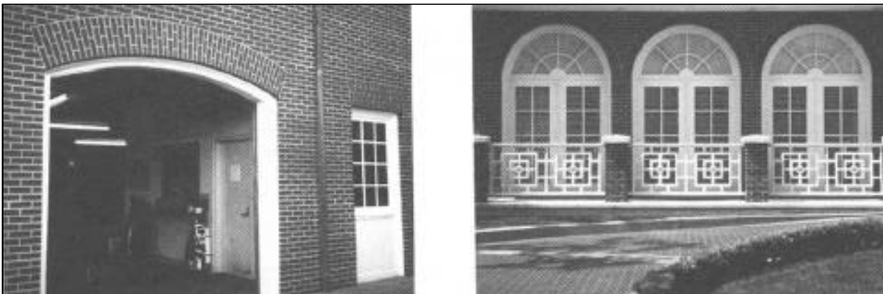
Structural Brick Arches FIG. 1
