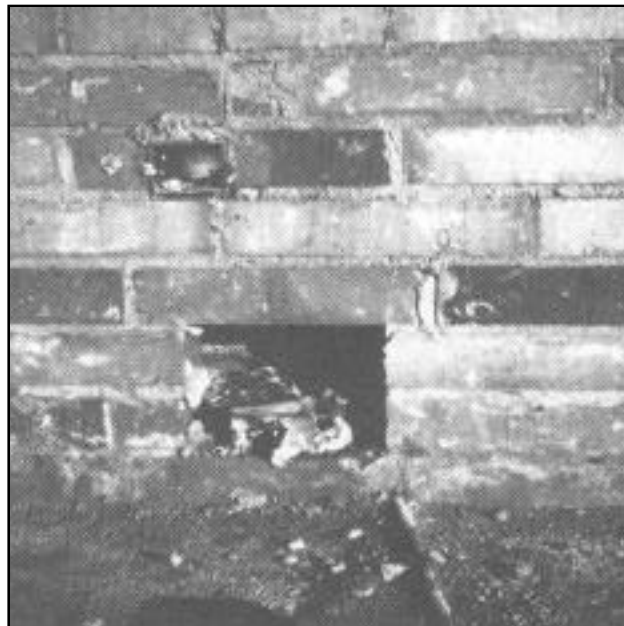
Grout Cleanouts FIG. 17
