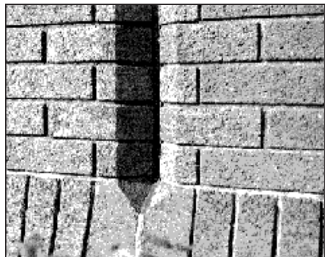
Accentuated Vertical Expansion Joint FIG. 16
